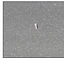
Finished mat with no warm mix additive
