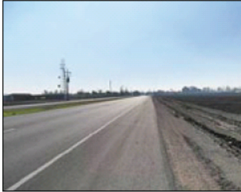
Airport Way: Paving with Sasobit warm mix additive
