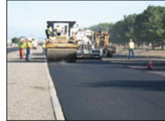
Paving with PG76-22TR
