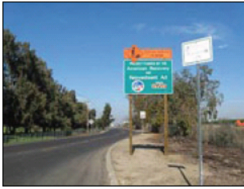
Manthey Road: Paving with Rediset warm mix additive.
